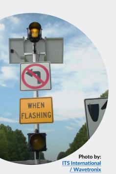
Intelligent Transportation Systems (ITS) companies, Applied Information and Wavetronix, announced a collaboration that has successfully piloted an early warning system in Peachtree Corners, Georgia. The system uses radar detection, advanced algorithms, and cloud computing to monitor the speed and trajectory of oncoming traffic and triggers a flashing beacon to warn turning vehicles of a potential conflict.
